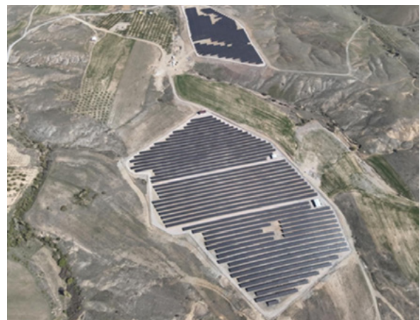
AISIN TURKIYE SOLAR POWER PLANT
