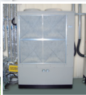
▼ Dual-mode heat pump system for use in production processes
