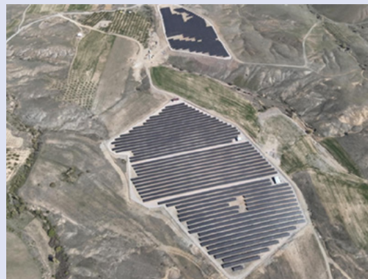
AISIN TURKIYE SOLAR POWER PLANT
