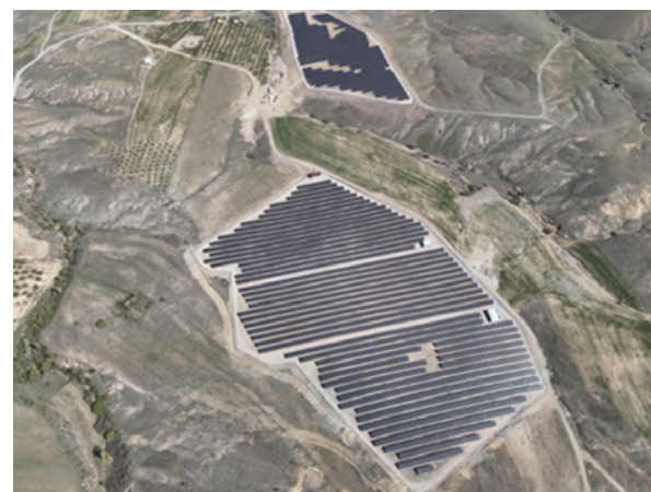
AISIN TURKIYE SOLAR POWER PLANT
