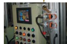
After installing the safety cover
